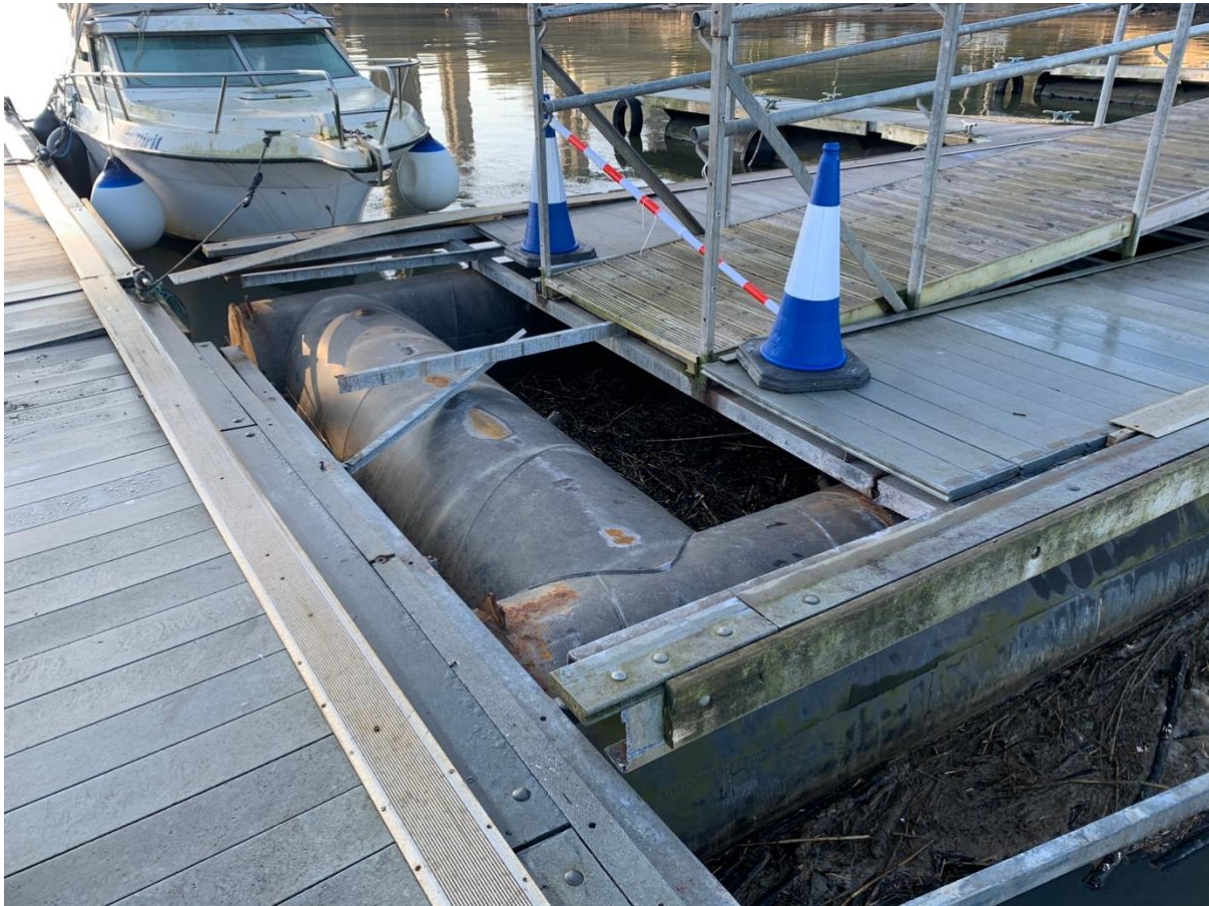
Damage at end of walkway pontoon
