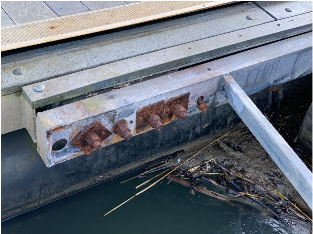
Corroded bolts on waterside pontoon join
