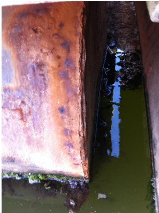
30m Pontoon Outer Tube North Corrosion & pitting on end welds
