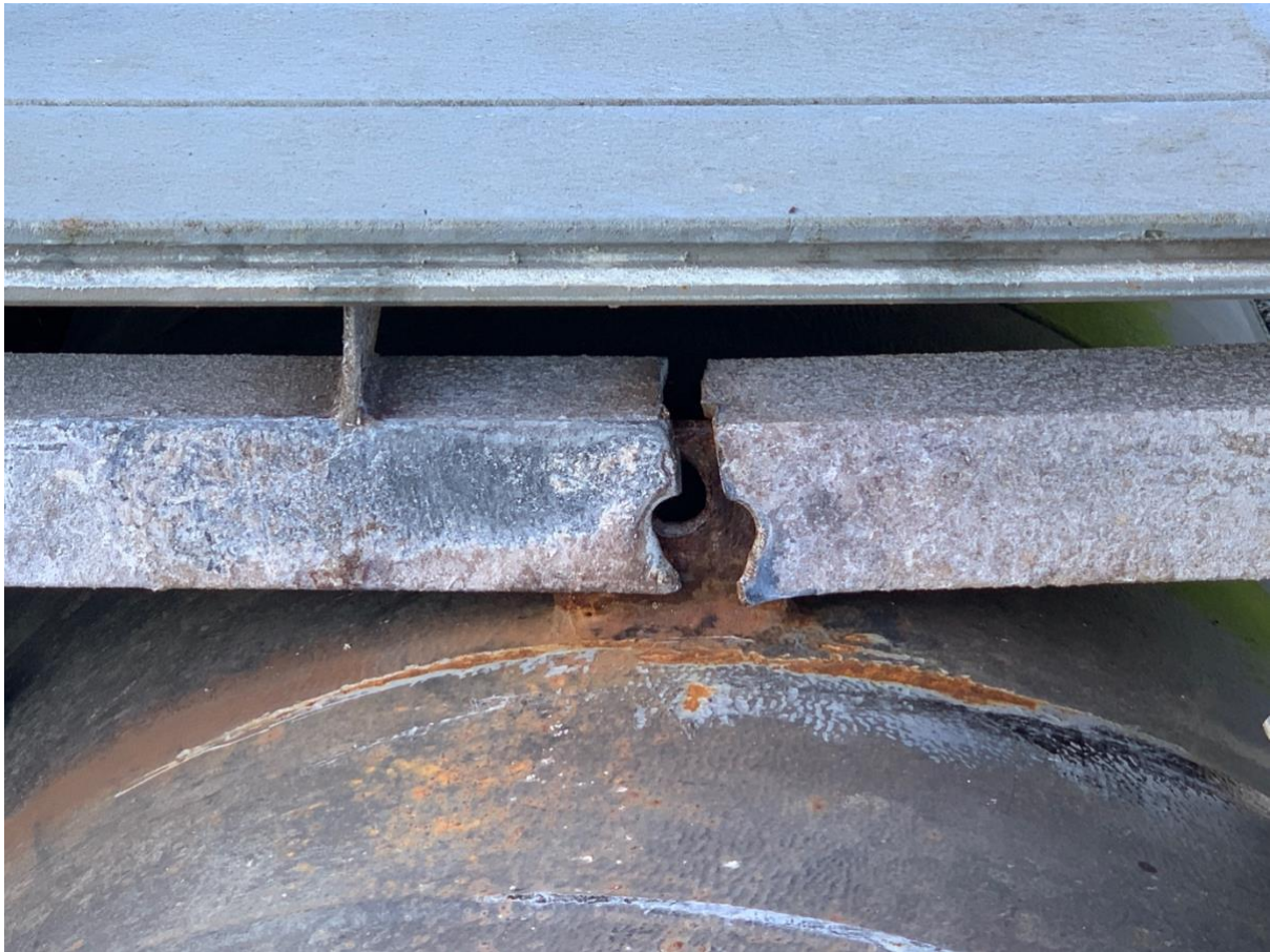
Broken float frame on walkway pontoon. Note the corrosion
