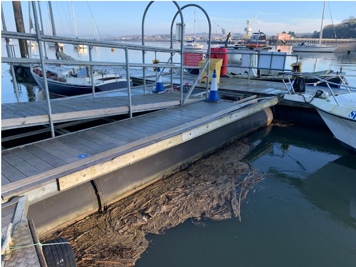
Walkway pontoon fouling
