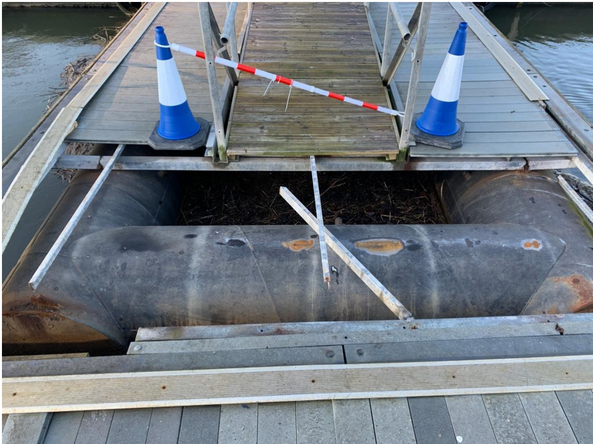
Damage at end of walkway pontoon
