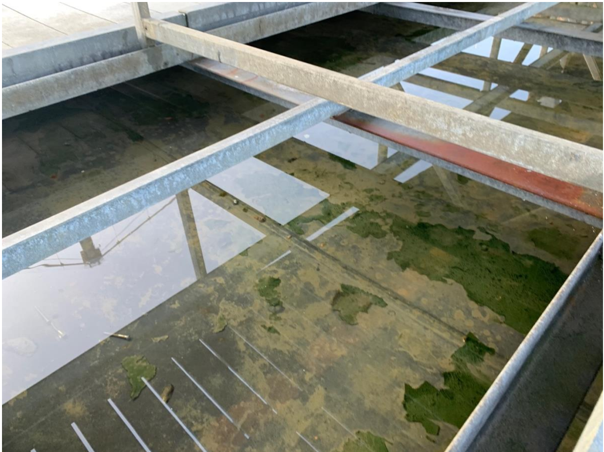
Water in top of walkway pontoon
